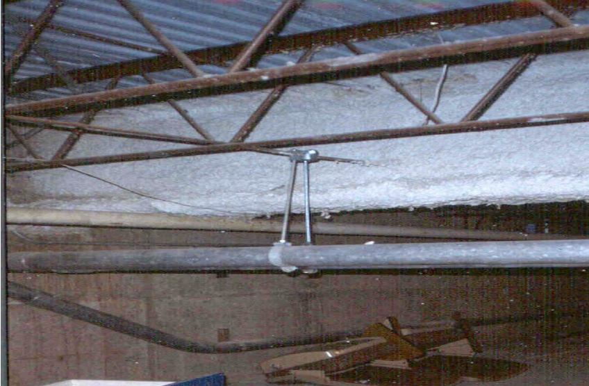
Example of friable asbestos - sprayed insulation
